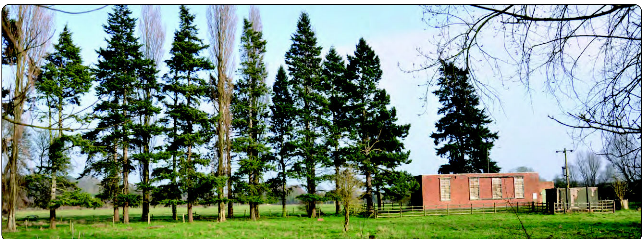
Photo F3. Eastern Pumping Station
