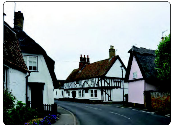
Photo B11. Houghton Manor Farmhouse
